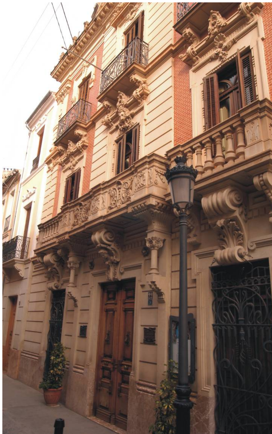
Main façade / Façana principal
